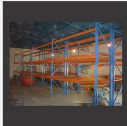
Pallet Rack Installation Service
